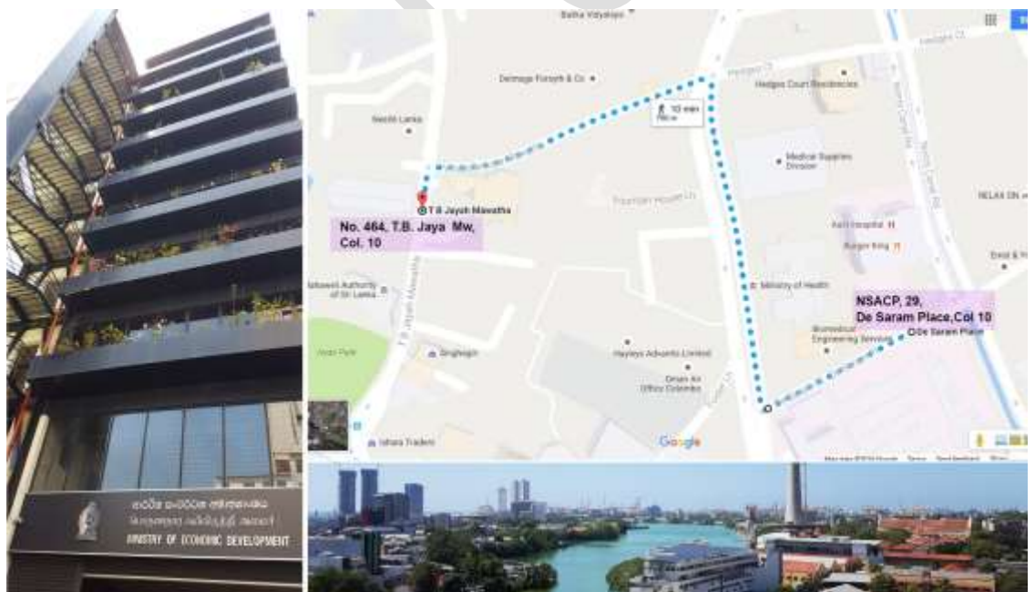
Figure 78: New building and its location map at No. 464, TB Jaya Mw., Colombo 10
